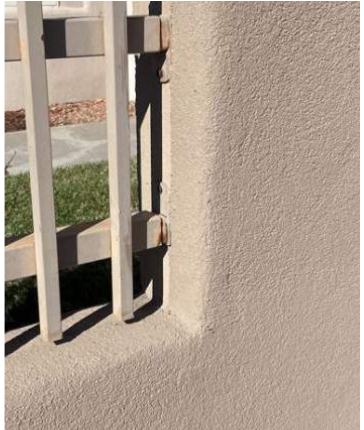
Attachment inserts allow expansion/contraction
